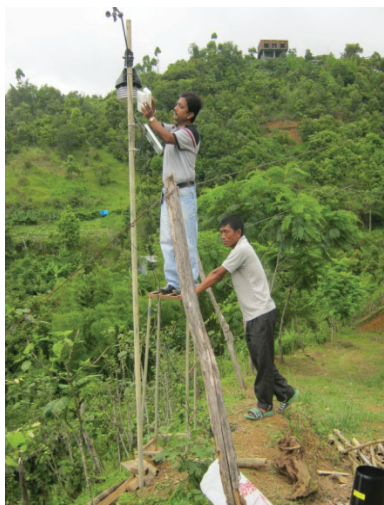
Installation of weather station in Vengsang Village
